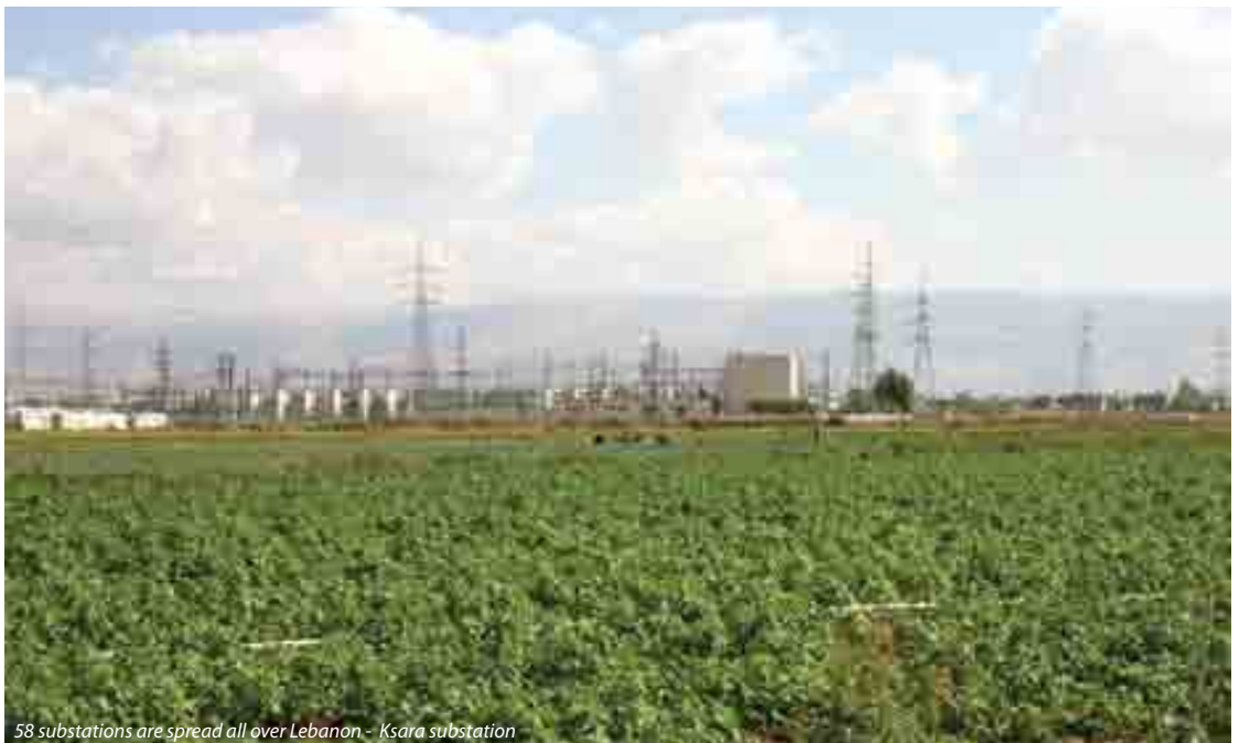
58 substations are spread all over Lebanon - Ksara substation
